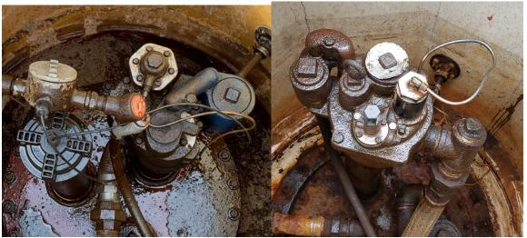
Sump components including fasteners, connectors, hardware, piping and leak detection equipment should be free of corrosion and material that interferes with inspection, maintenance and removal.
